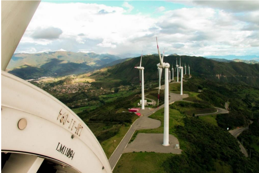
Figura 1.14. Central Eólica On Shore [92]
