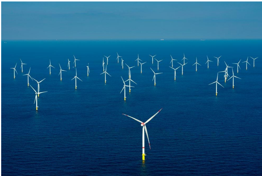
Figura 1.15. Central Eólica Offshore [96]
