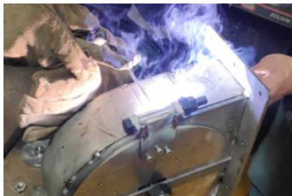
Figura 54. Bisagra soldada
