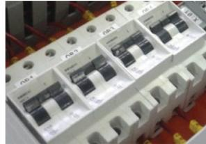
**Figura 2.9** Breakers termomagnéticos (QB1, QB2, QB3, QB4)
