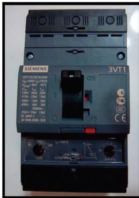
Figura 2.29: Breaker principal
