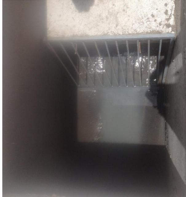
**FIGURA 4.2 REJILLA Y CANAL DE CRIBA DESPUÉS DE SU LIMPIEZA**
