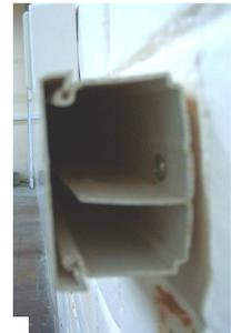
FIGURA 2.3: CANALETA INSTALADA
