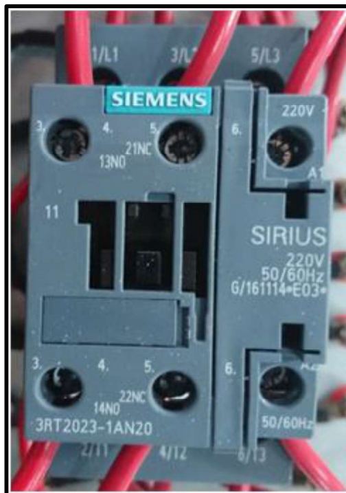
Figura 3.4 Contactor SIRIUS 3RT2023 AC-3, 4KW/400V, 1NO+1NC, AC 230V 50/60 HZ.
