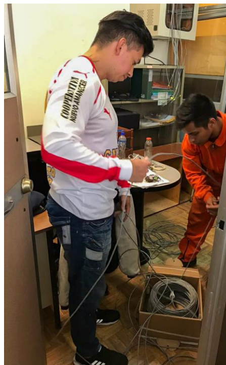
Figura 3.11: Cable UTP (5e)
