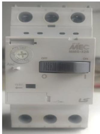
Figura 3.3 Guardamotor MMS-32S
