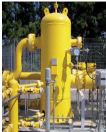
Figura 1.4. Knockout Drum vertical (API 520, 2008)
