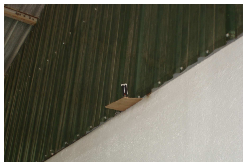
Figura 4-11: Antenas Wireless Bodega
