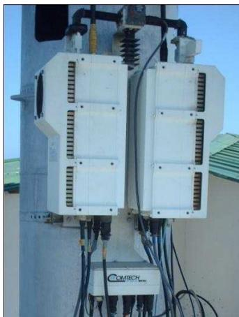
**Fig. 1.5 Transceiver 50 watts. Redundancia**
