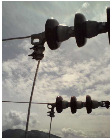
Figura 3.76 Conductor anclado
