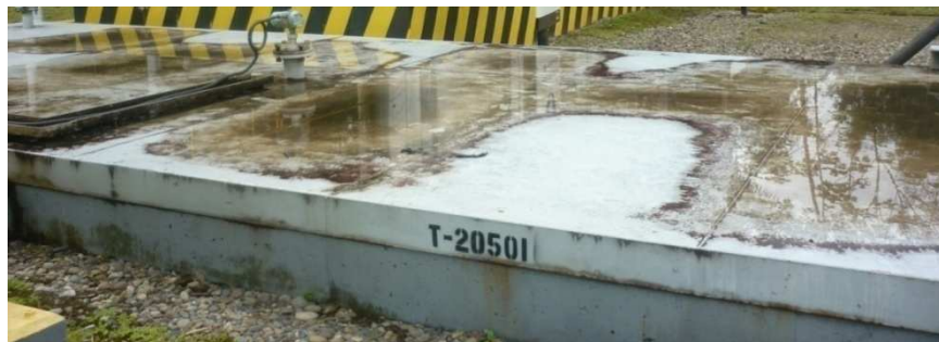
Figura 3.76: Tanque slop
