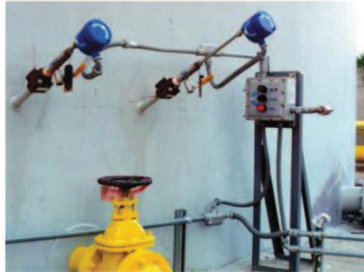
Agar ID System 1 & 2 Tank Installation
