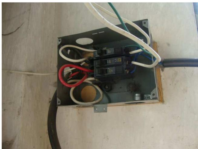
Figura 2.23 Interruptor tripolar termomagnético principal
