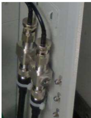
Figura 2.17 Lightning Arrester
